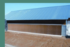
Cooling Pads & Fans
