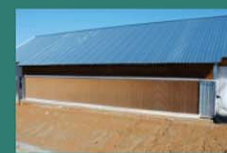
Cooling Pads & Fans
