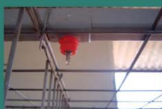
Nipple & PVC Pipe with Saddle
