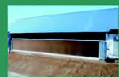
Cooling Pads & Fans
