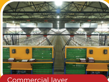
Commercial layer California cage systems
