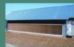
Cooling Pads & Fans
