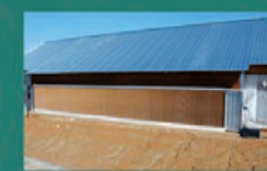
Cooling Pads & Fans
