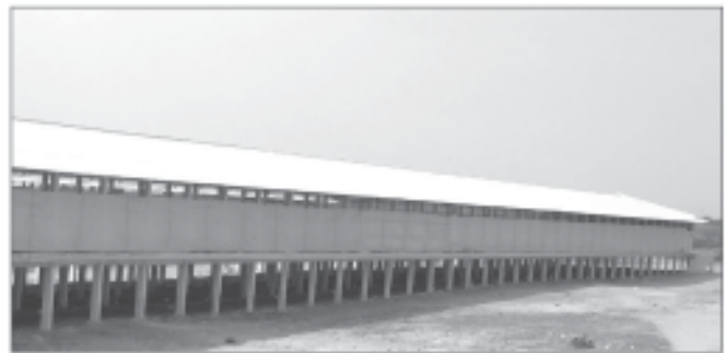
Figure 4. Lowering the curtain at the top creates better ventilation.
