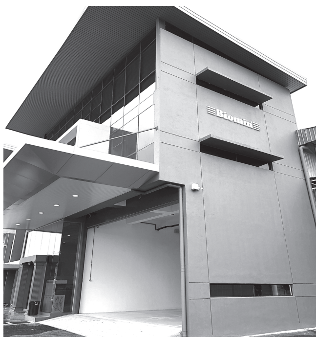
BIOMIN Malaysia Building
