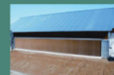
Cooling Pads & Fans
