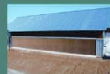
Cooling Pads & Fans
