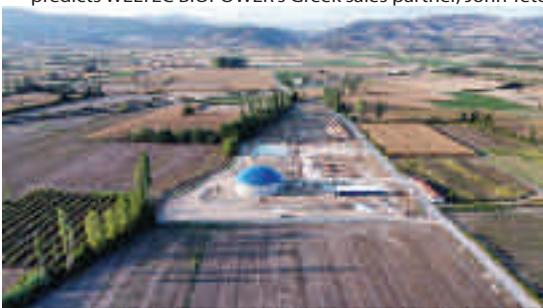
The Greek agricultural sector has trusted WELTEC BIOPOWER's biogas technologies since 2007 - and this trend is continuing. Most recently, three biogas plants were built, which the German manufacturer designed together with its Greek cooperation partner Tektoros Machinery.
